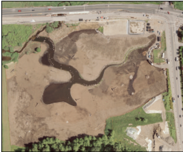
An aerial view of the mitigation site taken after construction in June 2007.
