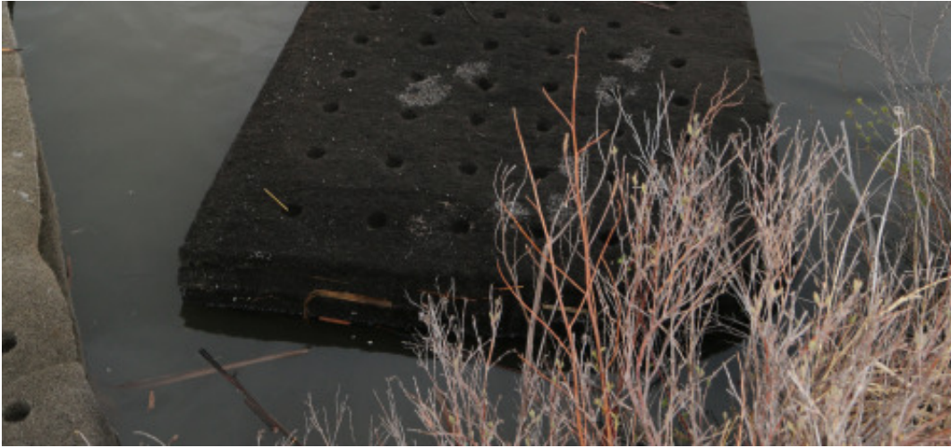
Half of the plastic base used for the floating island. Photo by Leith Edger / USFWS
